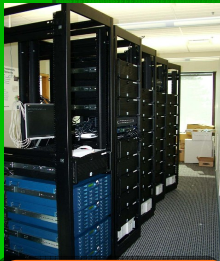
Fig 2: The RIT GRAPE cluster "gravitySimulator" is in operation since February 2005. Here are some of the technical details:
